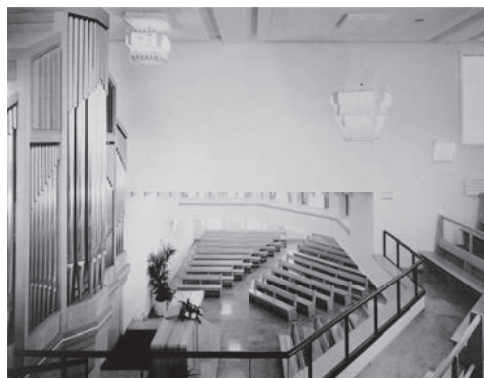
9 Neupostolische Kirche, Teff Sarasin, view of the church before the renovation.
